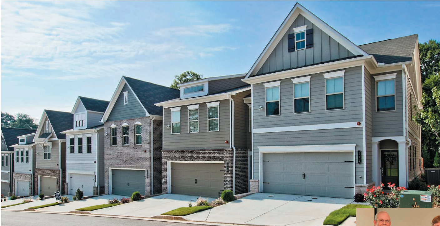
North Square, one of the many successful townhome communities Traton has built in metro-Atlanta over the past five plus decades.
